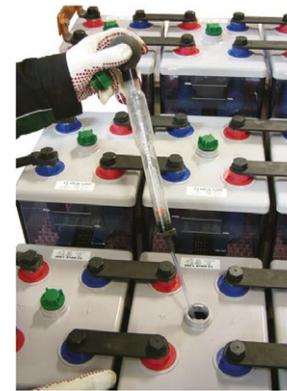
Fig. 6-2: Hydrometer
