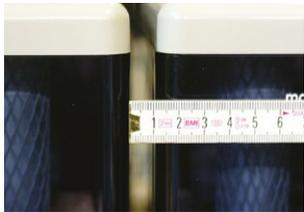
Fig. 5-13: 10 mm clearance between the batteries
